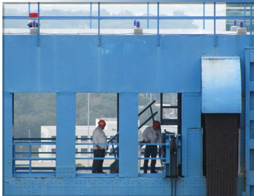
MAIN STREET BRIDGE INSPECTION
