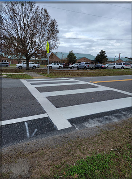
SCHOOL ZONE CROSSWALK IN DIXIE COUNTY
