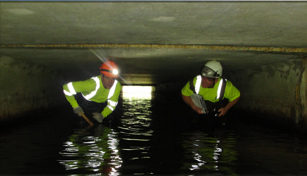
STRUCTURES MAINTENANCE CREW INSPECTS CULVERT
