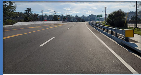
ALLIGATOR CREEK BRIDGE STRIPING
